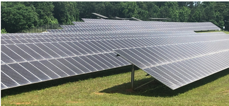
Fig 3. South-facing Arrays C and D (foreground) and south-west facing Array B (background). Arrays C and D generate more energy over an average day than B, but B generates more during periods of peak demand (early evening). The small shadows in this image indicate that the photograph was taken near to solar noon; in the early morning, the shadow would extend back towards, and even onto, the row behind.
