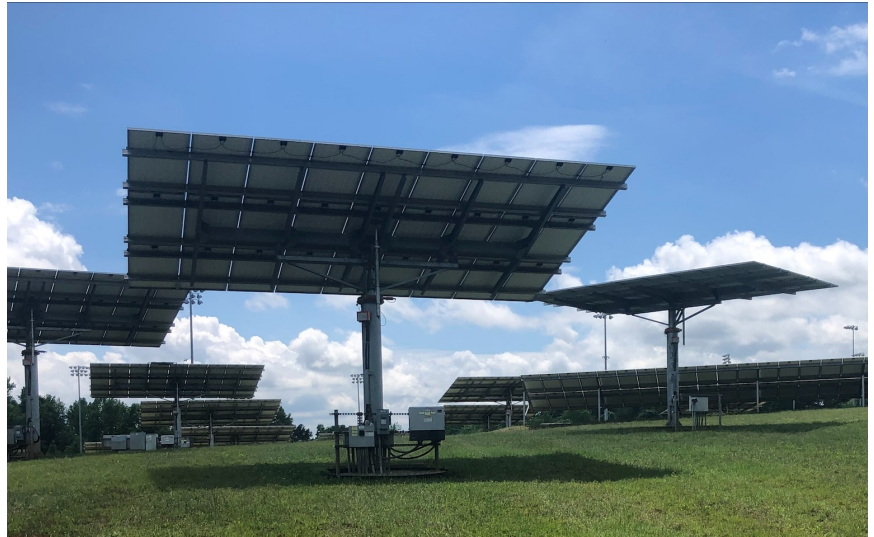
Fig 9: DAST—rear view. These modules are significantly larger in size, higher mounted, and further spaced, than SAST or fixed-angle trackers. The unit to the right is clearly at a flat angle, not tilted towards the solar zenith, indicating it has reverted to its default position due to a failure in its tracking system. DAST systems are most effective at high latitudes (where sun angle varies most) and where the availability space determines that a single, large, module is preferable to a longer row array.
