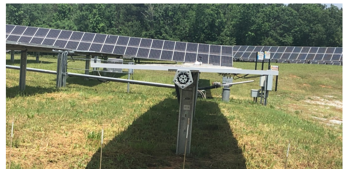
Fig 7: SAST- axial view. The pentagon-shape is the end of the rotational arm onto which the modules are fixed and which forms the axis of rotation. The hydraulics that rotate the module are visible, sticking out to the right, under the module. The array above/behind is the south-facing fixed array, the array to the right is the south-east facing array.
